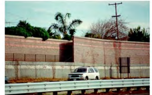
Figure 67. Noise wall behind cast-in-place retaining wall photo #1745
