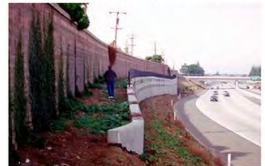
Figure 68. Noise wall behind cast-in-place retaining wall photo #1691
